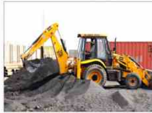
Machine : Excavators Company : JCB Escort Capacity : 20 Cum/Hr. Number : 06 Nos.
