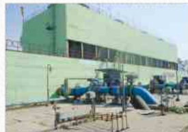
Petro Chemicals Buildings
