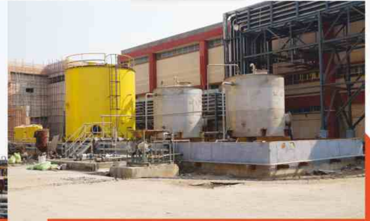
HCL AND H 2 SO 4 TANK FOUNDATION
