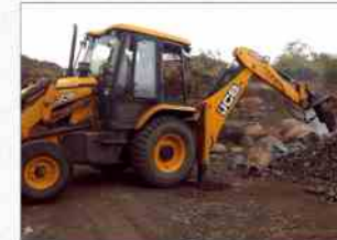
Machine : JCB Rock Breaker Company : Escort Number : 03 Nos.
