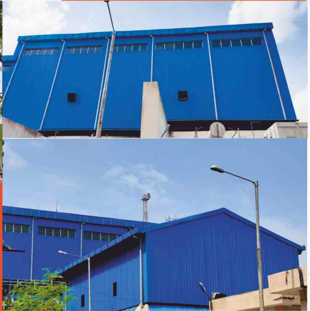
SANDWICH CLADDING, BY M/S. SNCLLP AROUND 5000 SQM
