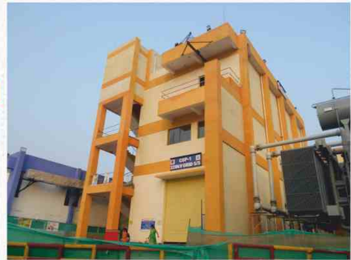
220KV GIS SUB STATION BUILDING
