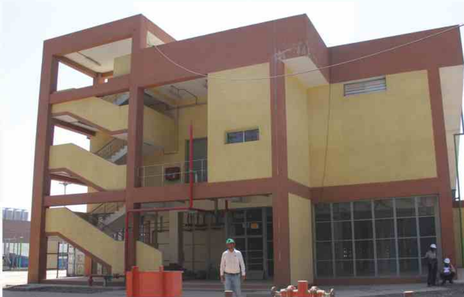
SUB STATION BUILDING
