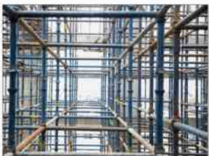
Machine : Shuttering Materials Company : Heavy For Industrial Use Number : 12000 Sqm. Remark : Propes, Jacks, Shuttering Plates, Cup lock Scaffolding System
